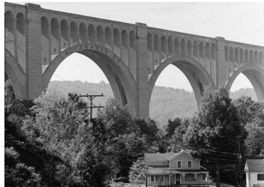
Figure 4. Tunkhannock Creek Viaduct
