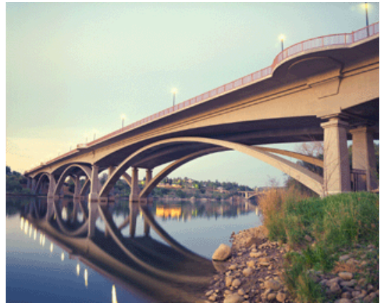
Figure 6. American River Bridge
